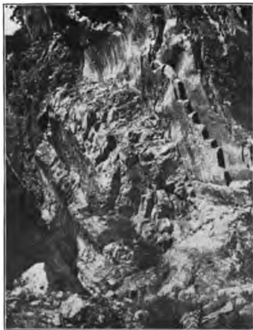
PLATE XXXIV(B).—Natural Cement Limestone Quarry in Elbrook Formation, One Mile East of Shepherdstown.
